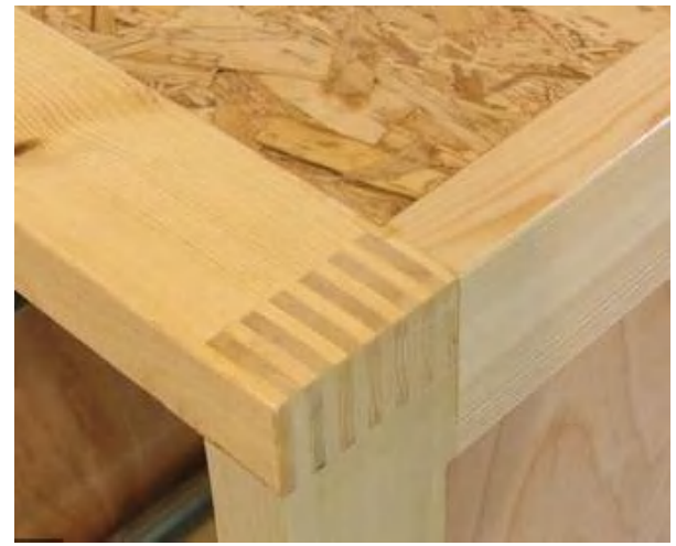
4. Solid wood corner joint
